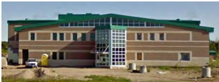
Photo 5-4: Queen Street Water Treatment Plant
