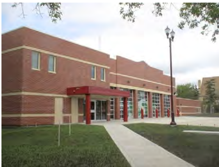
Photo 5-1: City of Yorkton Fire Hall
