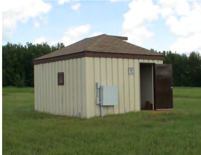
Photo 5-2: City of Yorkton Groundwater Pumphouse #10
