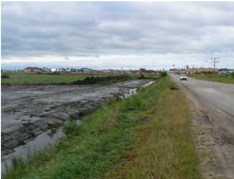
Photo 5-9: Dracup Avenue Storm Water Channel
