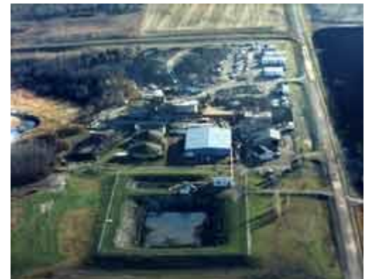
Current plant under construction. 1990
