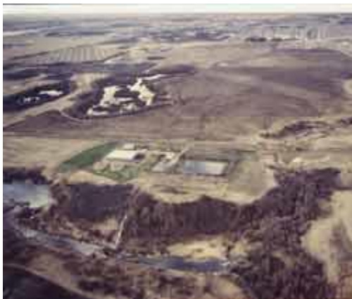
Aerial view of the second mechanical plant and lagoons. 1982
