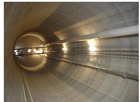
Vertical view of the interior of the water tower shaft.
