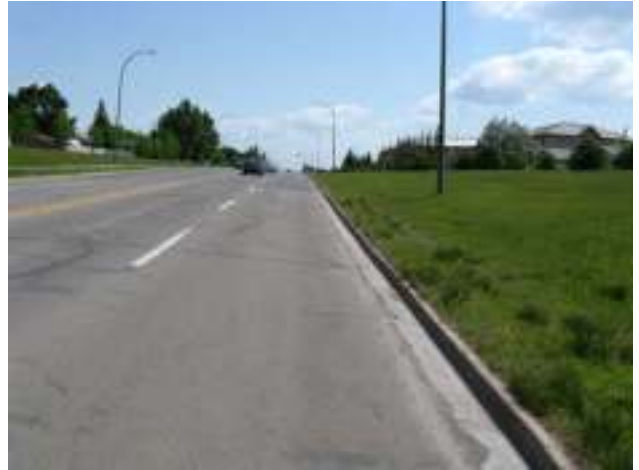
Photo 50: Darlington Street East Looking West (West Bound Lane) of the Overpass with No Sidewalk
