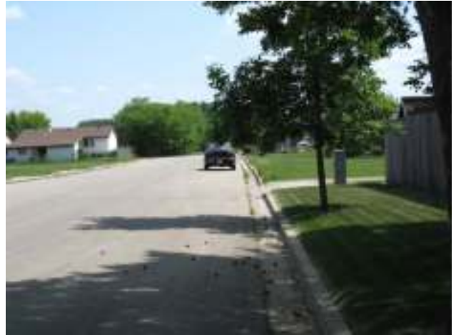
Photo 32: Henderson Street East Looking West
