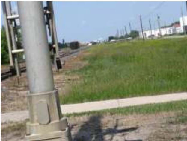
Photo 39: Sidewalk at the Intersection of Smith Street
