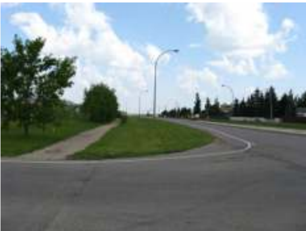
Photo 57: Mayhew Ave & Fietze Street Looking North
