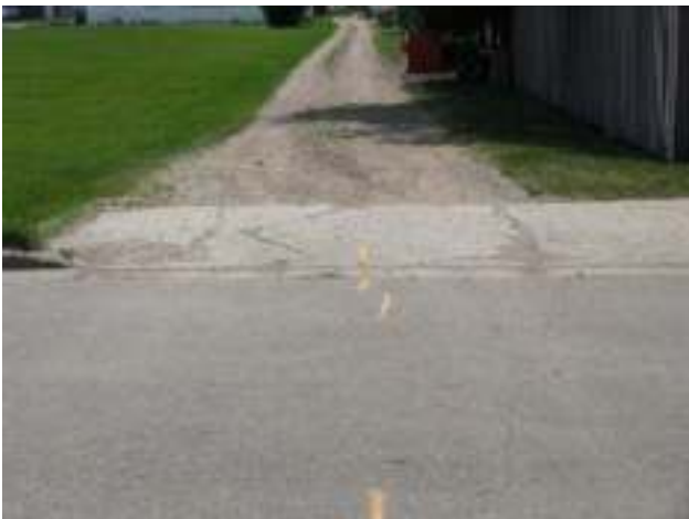
Photo 33: Granular Pathway Intersecting Henderson Street Looking South
