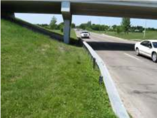
Photo 49: Darlington Street East Looking East Under the Overpass. Note: No Sidewalk
