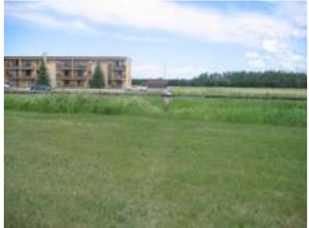
Photo 20: Work Foot Path Across Railway Tracks East of Sunset Drive
