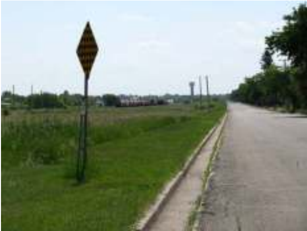
Photo 37: Victoria Avenue Along Rail Tracks
