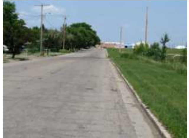
Photo 38: Victoria Avenue North Bound Lane Parallel to the Train Tracks
