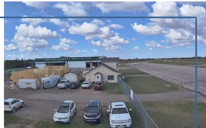
Airport Terminal Building
