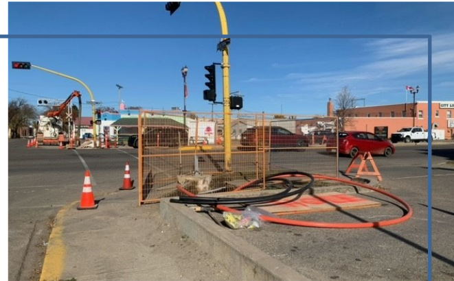
Traffic Signal Pole Replacement
